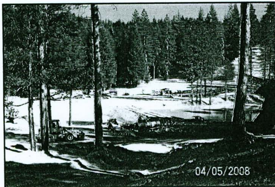
Photo 6. Photo looking east across staging area.
