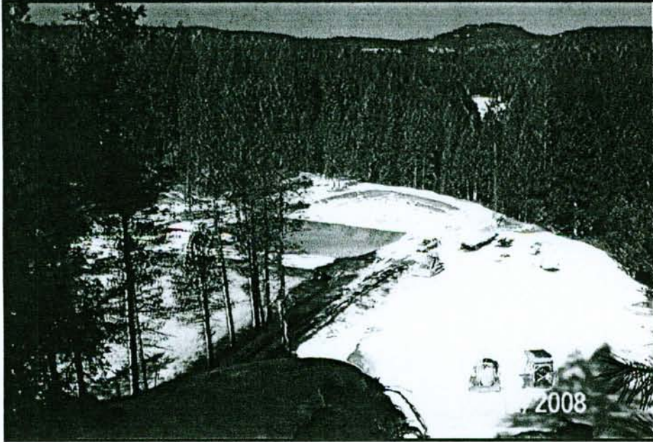
Photo 1. Photo looking north with the ponds and staging area. Greenhorn Creek is in the background.
