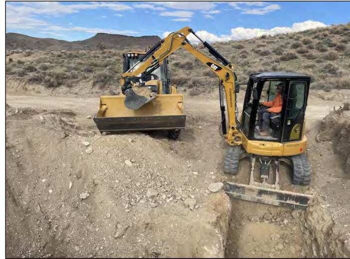
Photos 11 B Digging out a crack in Trench T-2.
