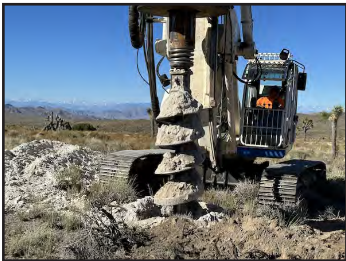
Photo 15 A. Drilling through the volcanic air fall ash.
